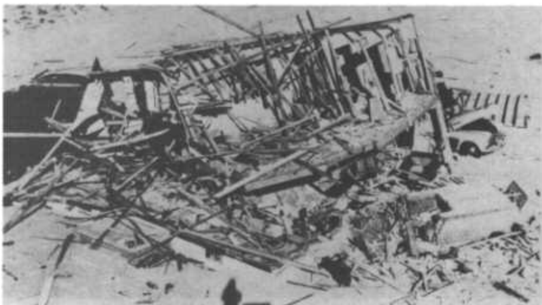
Fig. 7.4. Unburned wreckage of the same two-story, wood-frame house pictured in Fig. 7.1 after being wrecked by the 5-psi blast effects of a small nuclear test explosion.
