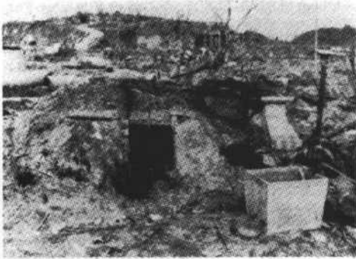
Fig. 1.5. Undamaged earth-covered family shelter in Nagasaki.
